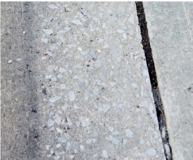
← Diamond Grinding and Diamond Sawing have the same effect on the Concrete surface, exposing the aggregate as clearly seen in these photographs.
